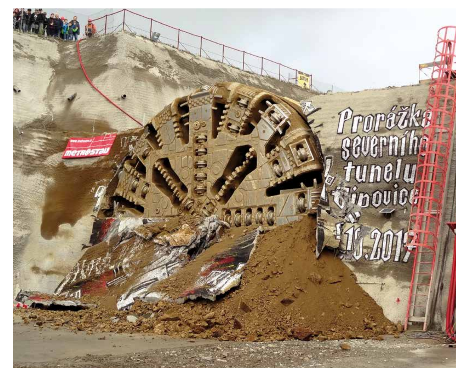
Prorážka severního tunelu Ejovice Breakthrough of the Ejovice northern tunnel, the Czech Republic
