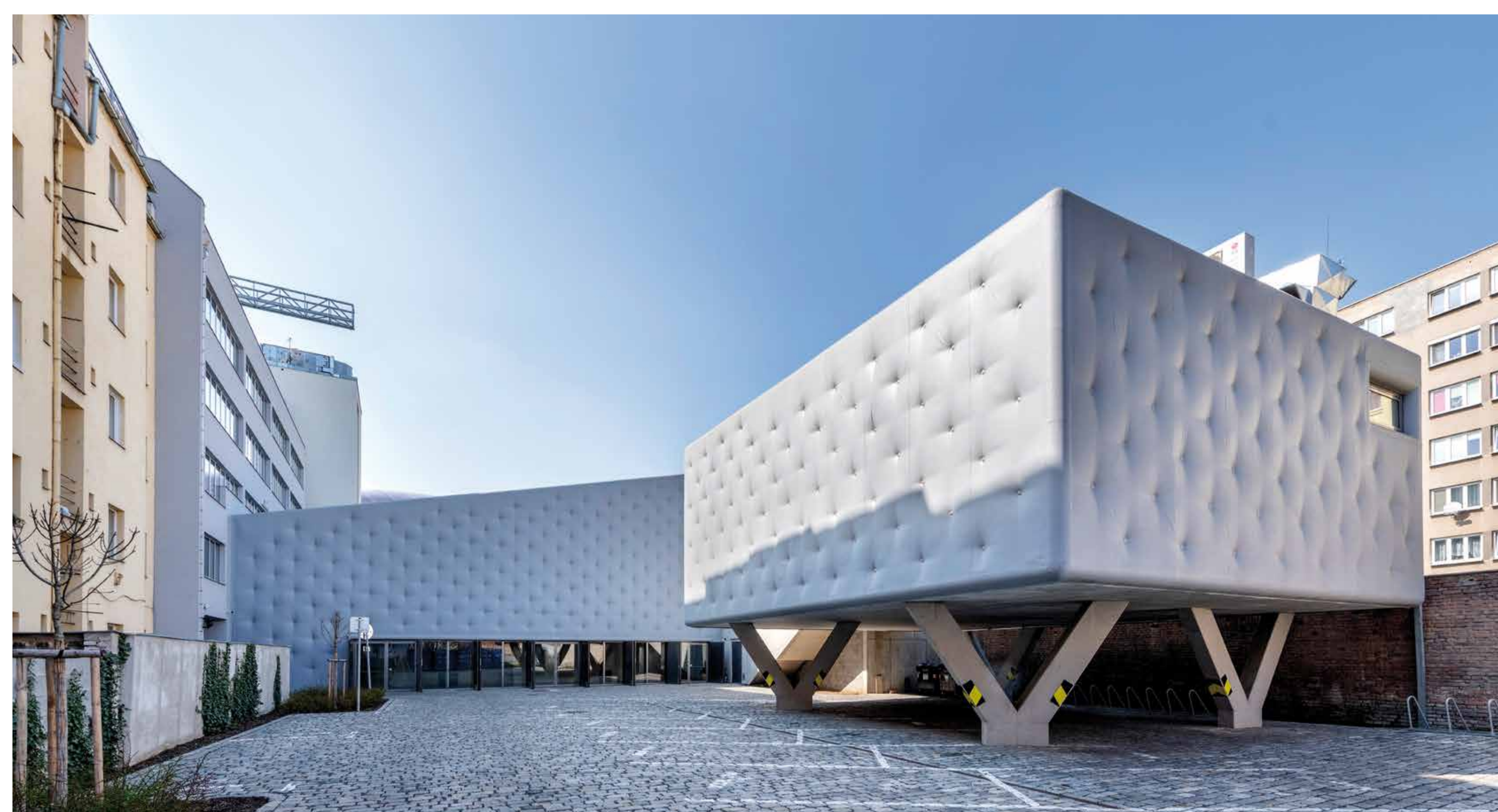
Centrum moderního umění NEW DOX, Praha NEW DOX – the extension of the Center for Modern Art, Prague, the Czech Republic
