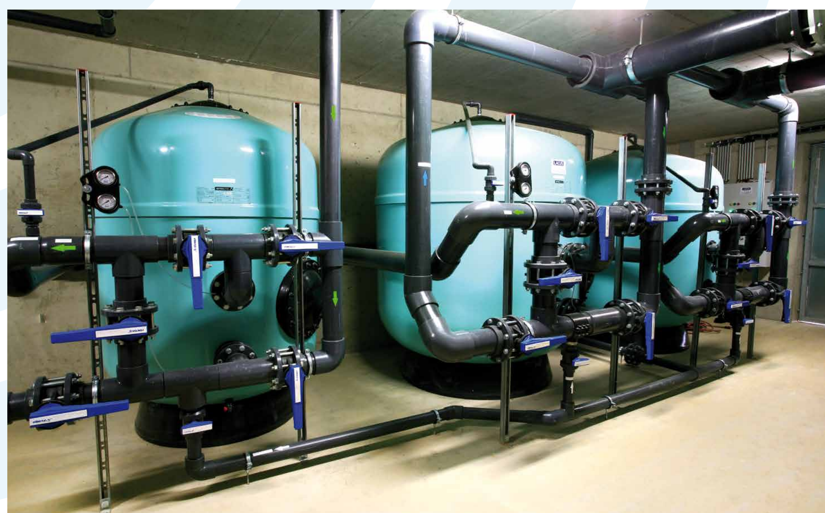
Písková filtrace v úpravně bazénové vody na koupališti v Kolovratěch Sand filtration in the swimming pool water treatment plant; the outdoor swimming pool in Kolovraty, the Czech Republic
